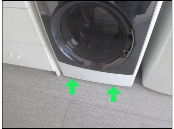
No Drip Pan On Main Floor Laundry
