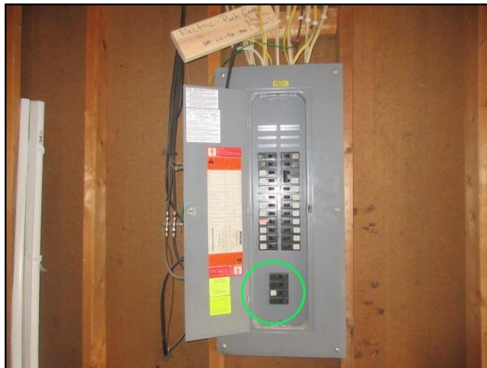
Main Electrical Shut Off
