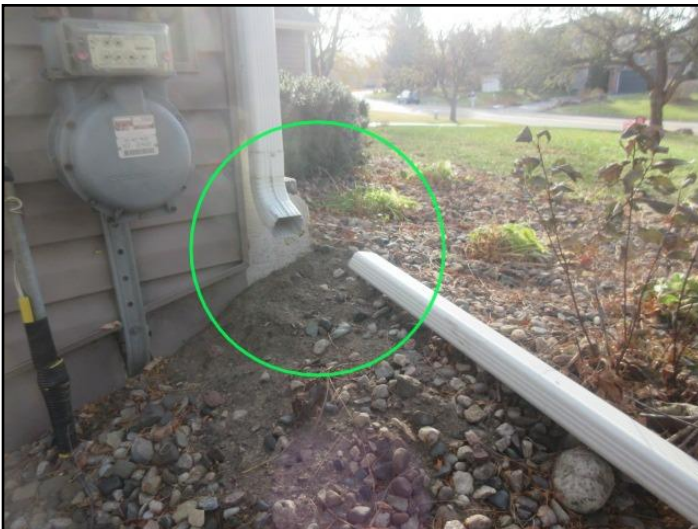
Disconnected Rear Extension
