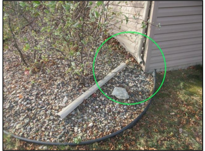
Disconnected Rear Extension
