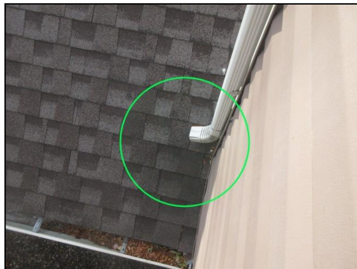
Discharge Onto Roof
