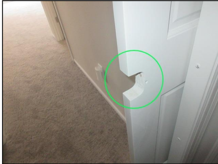
Entry Pocket Door Missing Hardware
