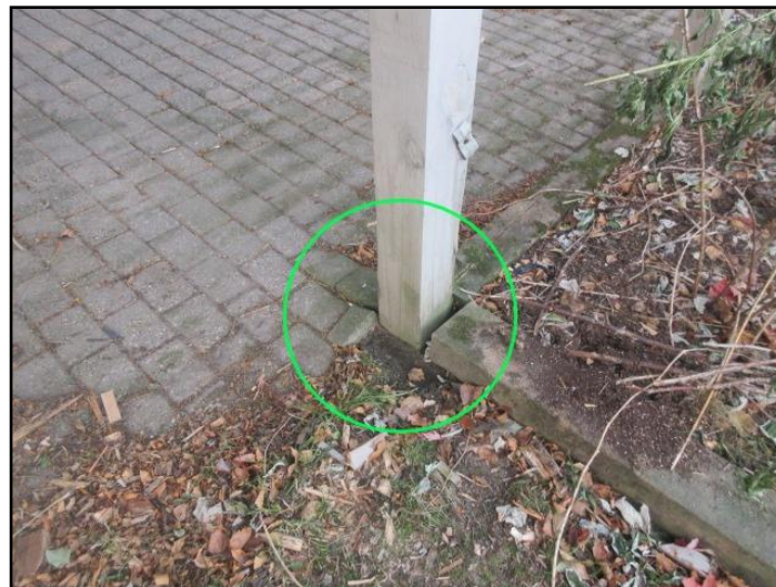
Deck Posts Appear Poured In Place
