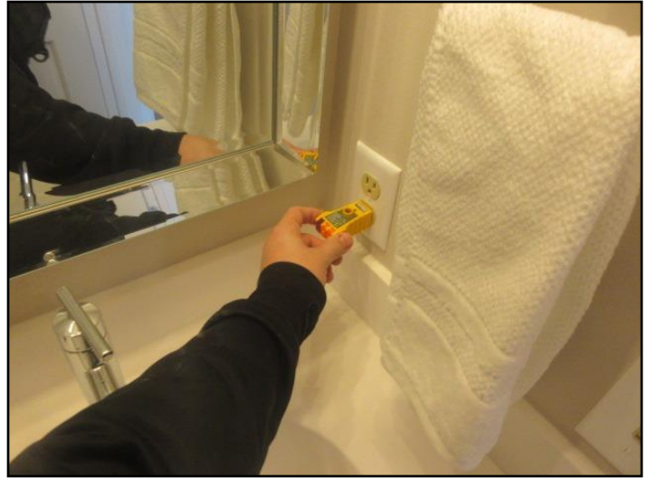
Loose Main Floor Bath Outlet
