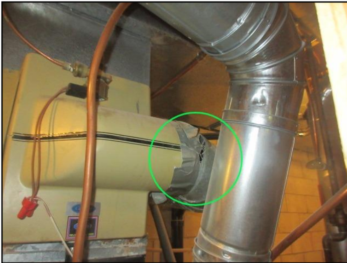
Poor Connection On Humidifier
