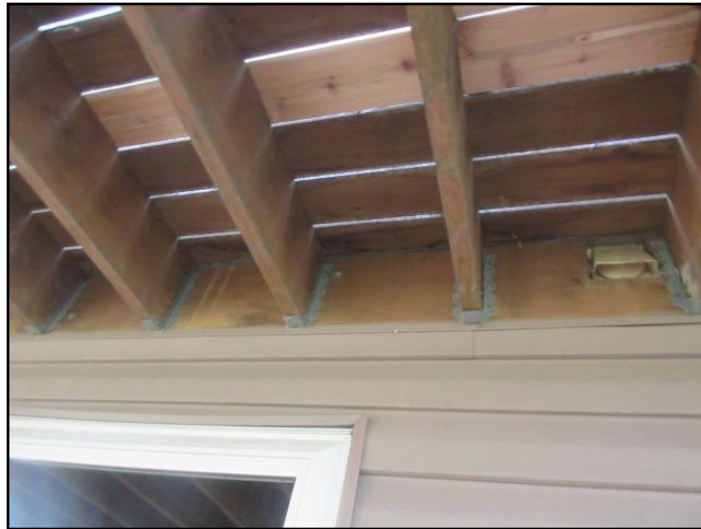
Joist Hangers And Flashing Present
