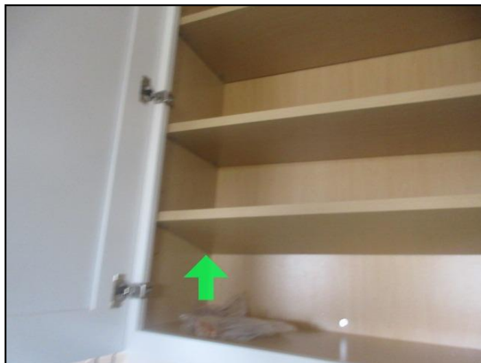
Missing Cabinet Bracket
