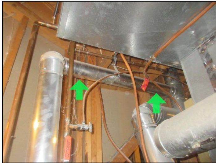
Water Heater Venting
