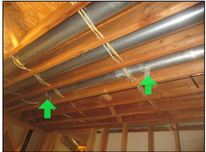
Duct Tape On Joints
