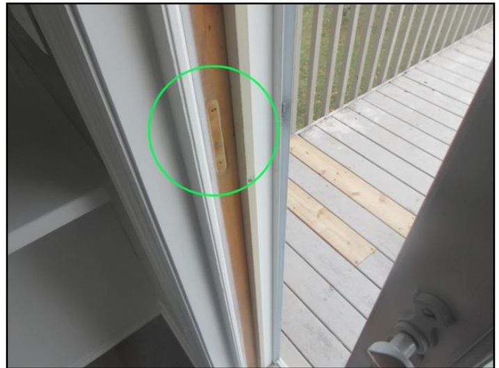
Main Level Patio Missing Lock Strike Plate
