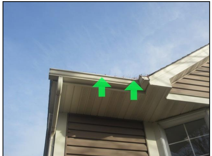
Gutters W/ Debris Front Exterior
