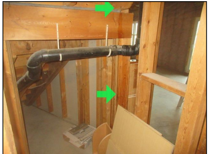
Leaking Followed Through Into Bsmt.
