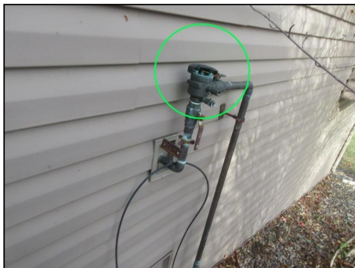
Back Flow Preventer Cap Damaged
