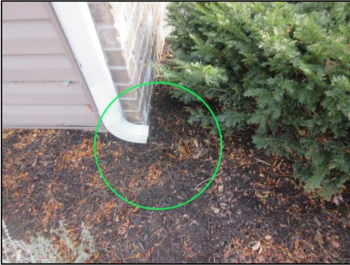
Missing Extension Front
