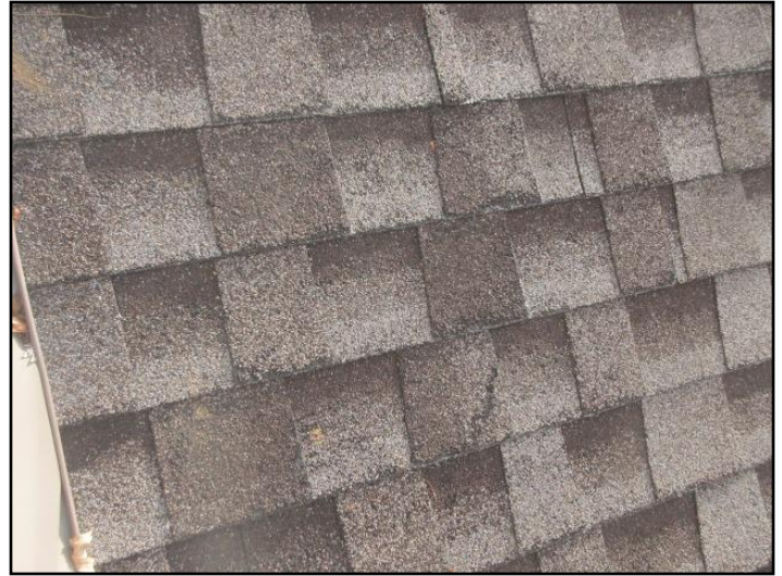
Some Granular Loss On Cosmetics Of Aging
