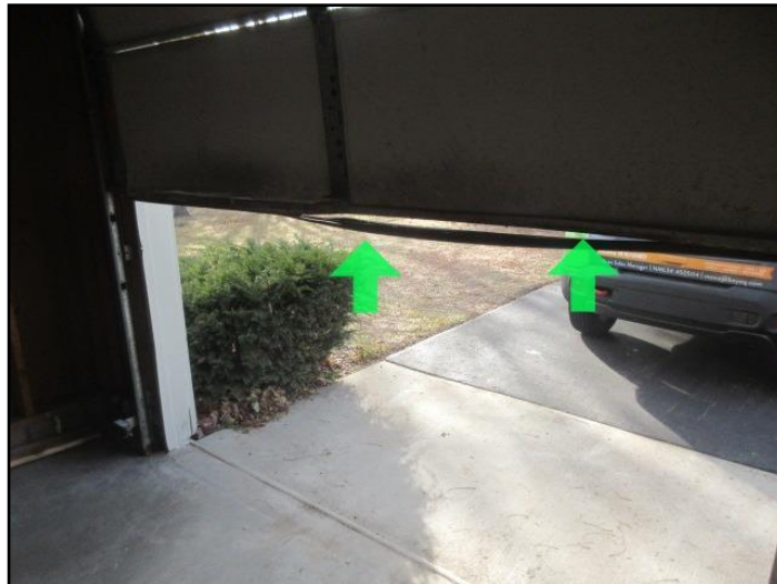
Failing Weather Stripping
